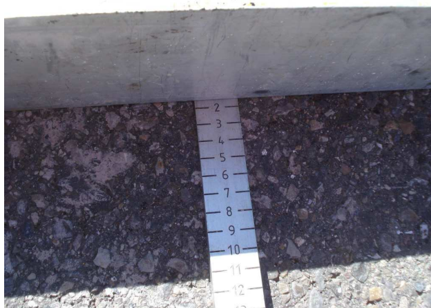
figure 8: ruts section C, L 181
