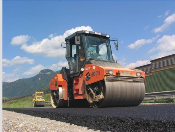
S35 Murtal Schnellstraße - km 27,5 - km 23,8, RFB Bruck/Mur, built in 2008
