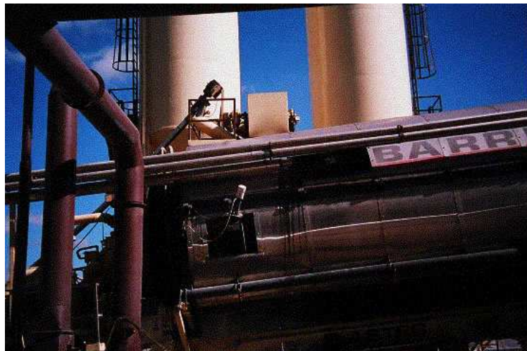
Figure 28: Asphalt plant in Georgia with two silos: one for mineral filler and the other for hydrated lime (from [145]).
