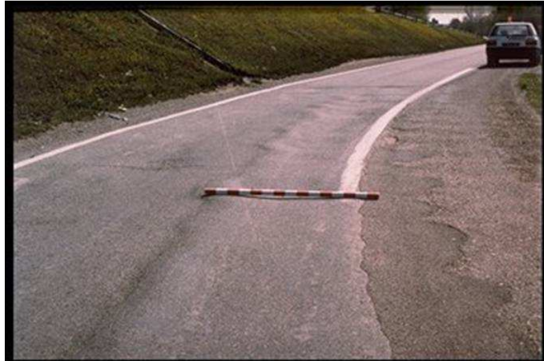
Figure 15: Rutting in an asphalt mixture (from [45]).
