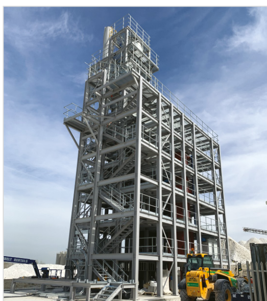
Zero-Carbon Lime pilot plant in final stages of construction (April 2022).
