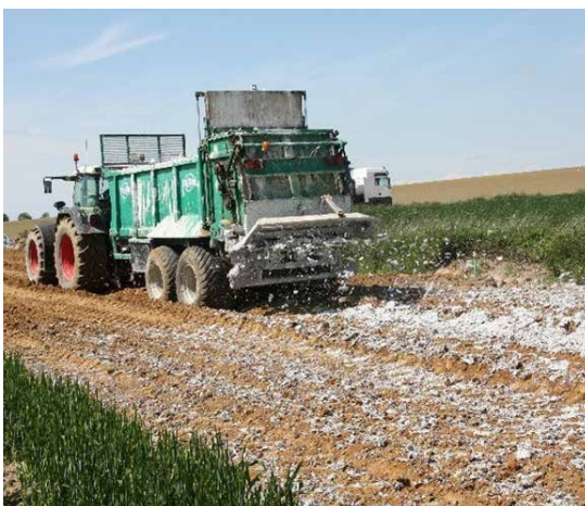
Figure 7.16 – Before and after treatment; lime spreading (© Nonet)
