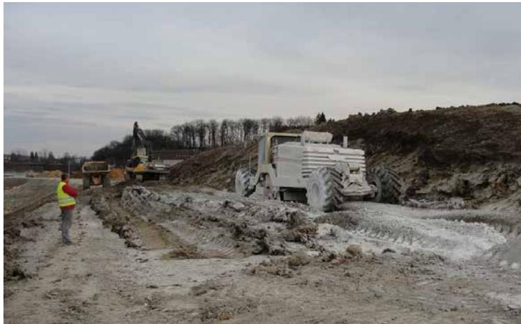
Figure 7.21 – Soil treatment operations (© Terdouest)
