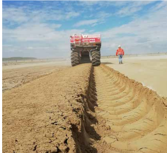
Figure 4.15 – Mixing – Pulvimixer (© Carmeuse)
