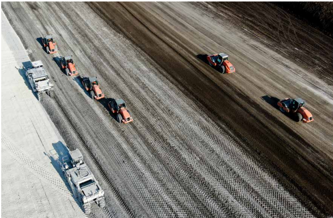
Figure 4.23 – Mixing and compaction operations (© Carmeuse)
