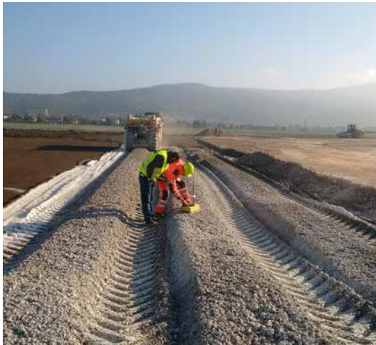
Figure 4.27 – Control of moisture, density, compaction ratio by nuclear gauge (© Carmeuse, BRRC)
