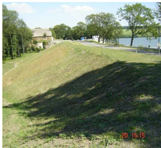
Figure 7.15 – Reconstruction of the 15 m high protection dyke at Hvezda (Czech Republic) using lime treatment of the sediments, after the floods of 2002 (© Lhoist)
