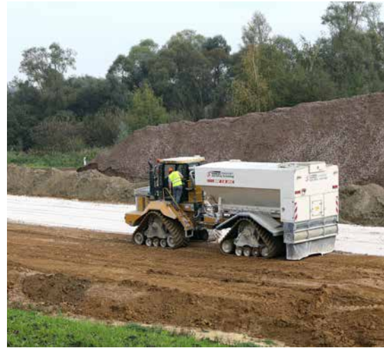
Figure 4.9 – Towed lime spreader (© Lhoist)
