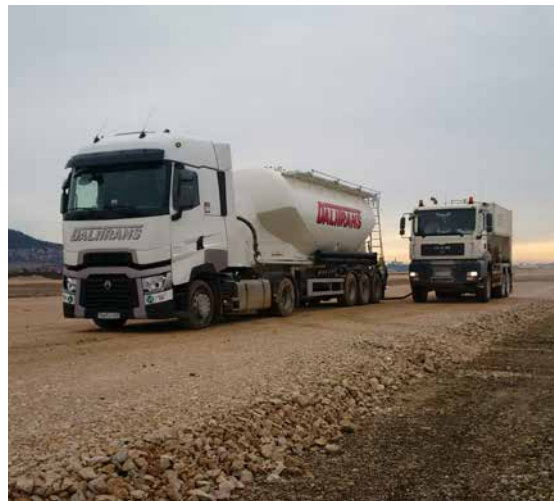
Figure 4.3 – Loading of spreader (© Carmeuse).
