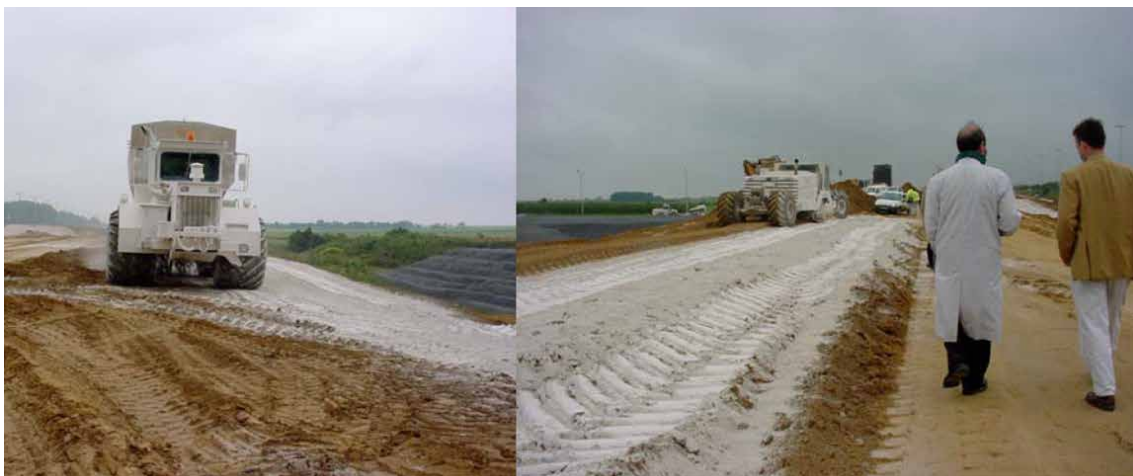
Figure 7.2 – Lime treatment on HSR sites (© Lhoist)
