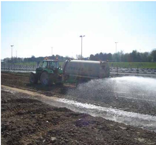
Figure 4.6 – Water addition to the surface before lime addition (© Lhoist)
