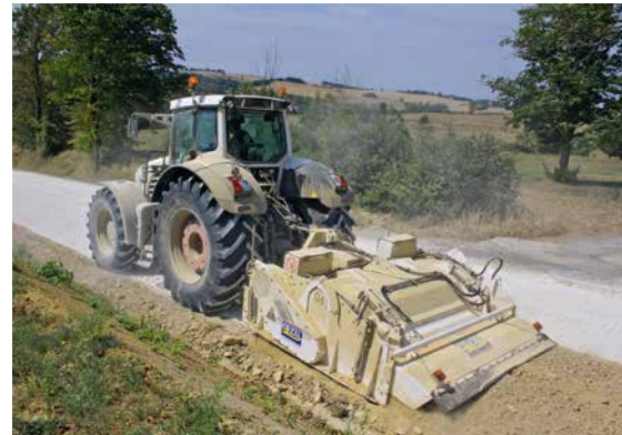
Figure 1.5 – Tractor-towed stabilisers for use in small-scale soil stabilisation projects (© Wirtgen)
