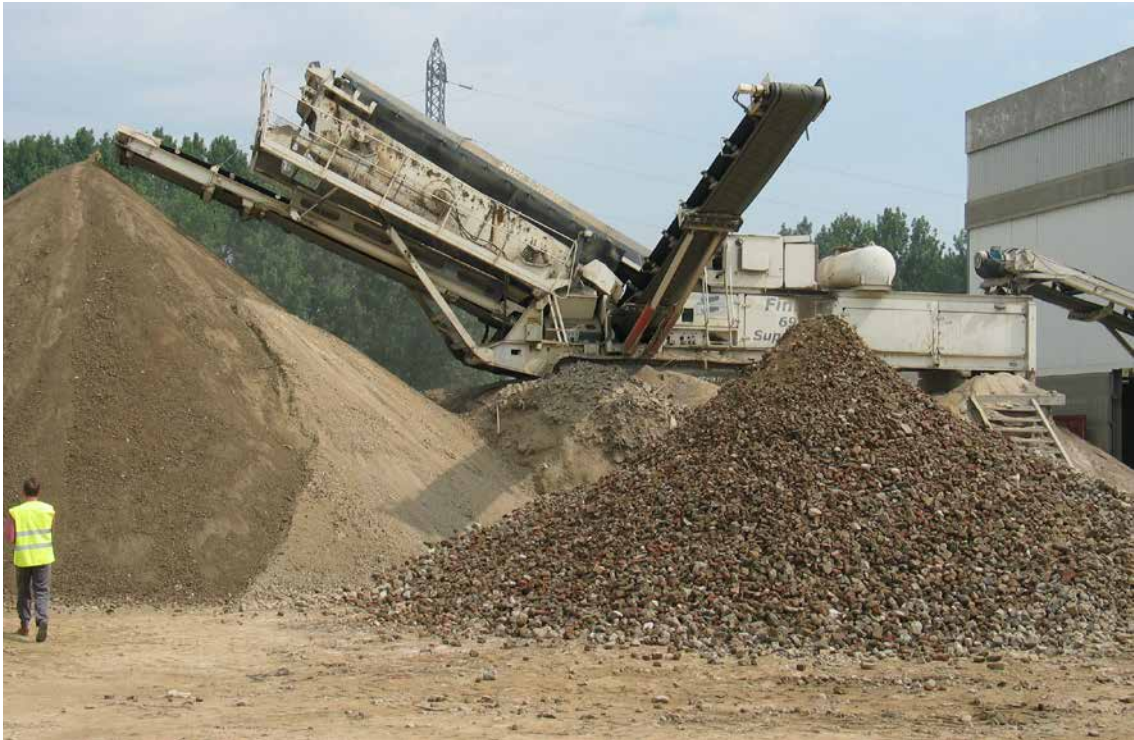
Figure 7.28 – Recycling platform (© Lhoist)
