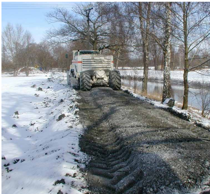
Figure 7.9 – Lime treatment in cold conditions (© Lhoist)
