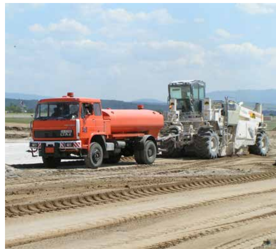
Figure 4.20 – Pulvimixer pushing water silo truck (© Carmeuse)
