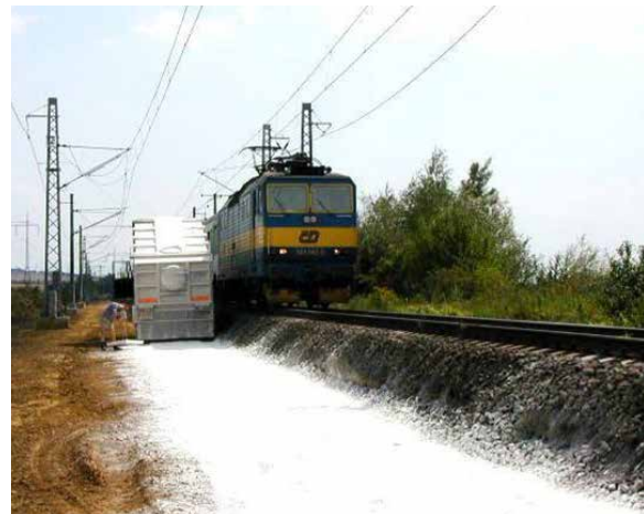
Figure 7.5 - Lime treatment on railway structures (Puiatti, D. & Robinet, A., Georail 2011)
