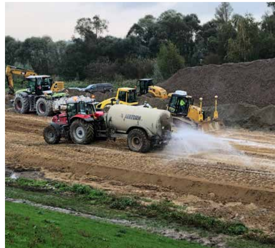
Figure 4.7 – Water addition to the surface before lime addition (© Lhoist)
