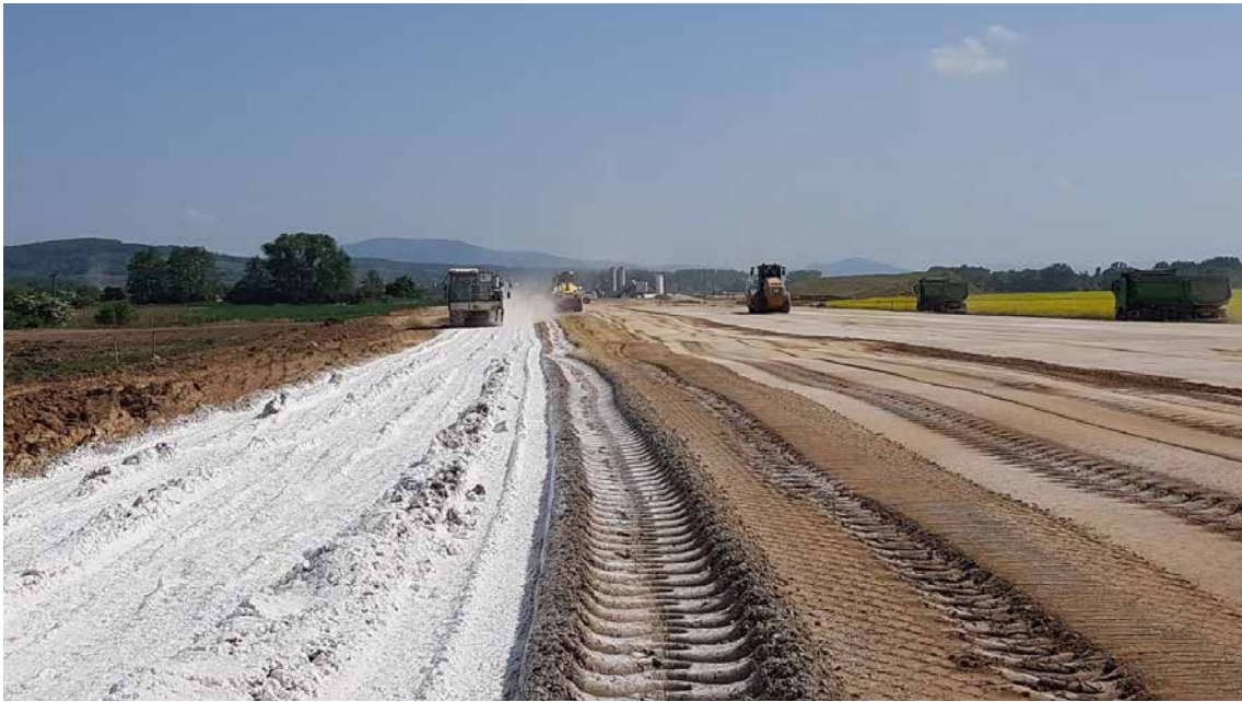
Figure 7.23 – Picture from a job site (© Carmeuse)
