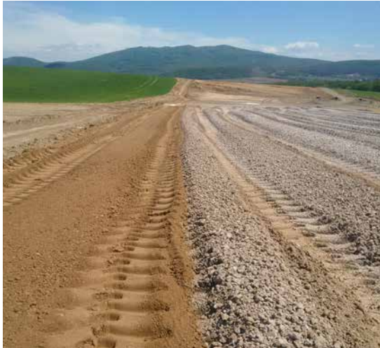
Figure 4.14 – Mixing operations (left two passes – right one pass) (© Carmeuse)
