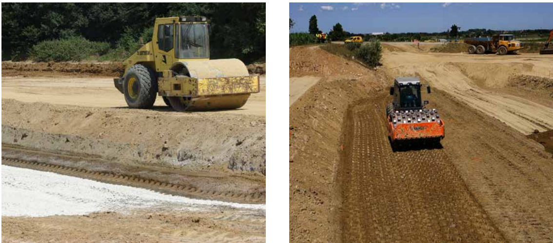
Figure 4.22 – Smooth drum roller / Padfoot rollers (© Lhoist)
