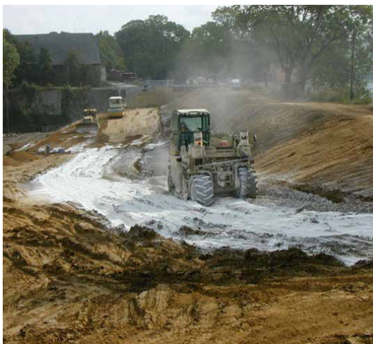
Figure 7.15 – Reconstruction of the 15 m high protection dyke at Hvezda (Czech Republic) using lime treatment of the sediments, after the floods of 2002 (© Lhoist)
