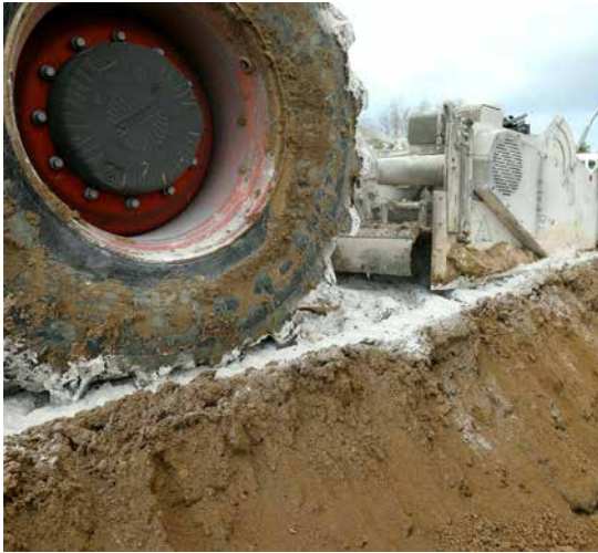
Figure 4.18 – Tractor-towed stabiliser (© Lhoist)
