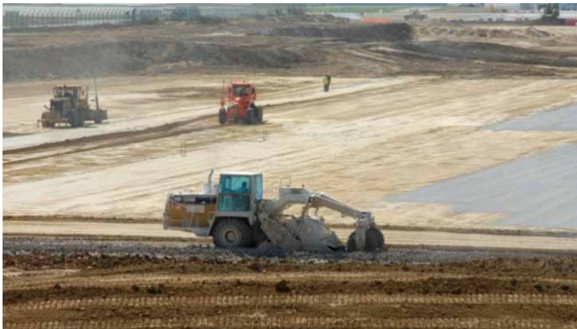
Figure 7.12 – Earthworks at Paris-Charles de Gaulle airport (Raynaud et al., 2008)
