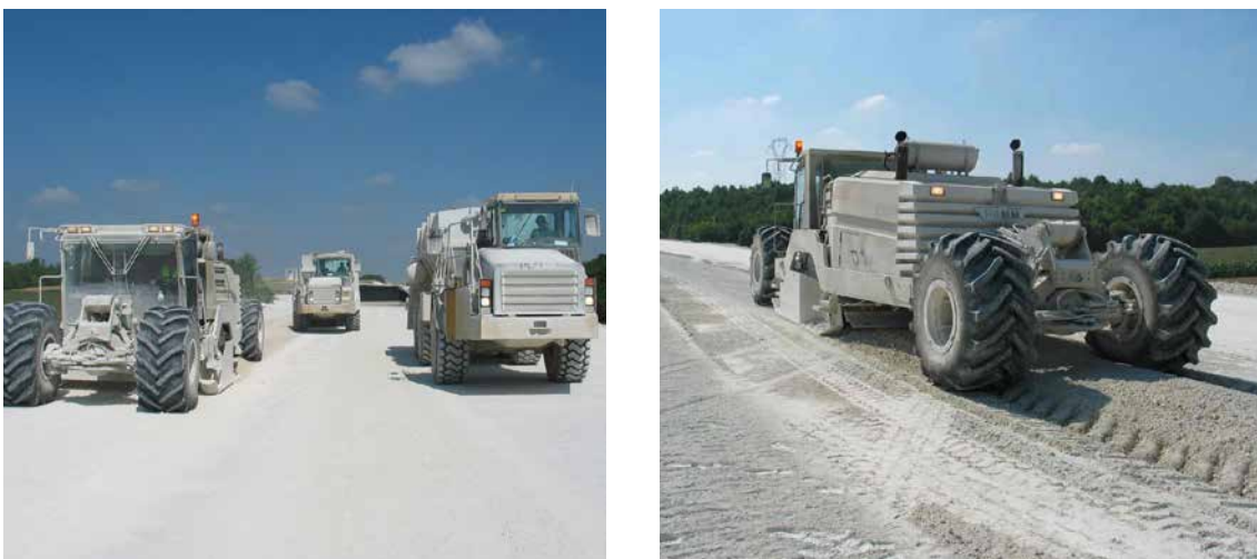
Figure 7.25 – Chalk treatment - TGV Est job site (© Lhoist)
