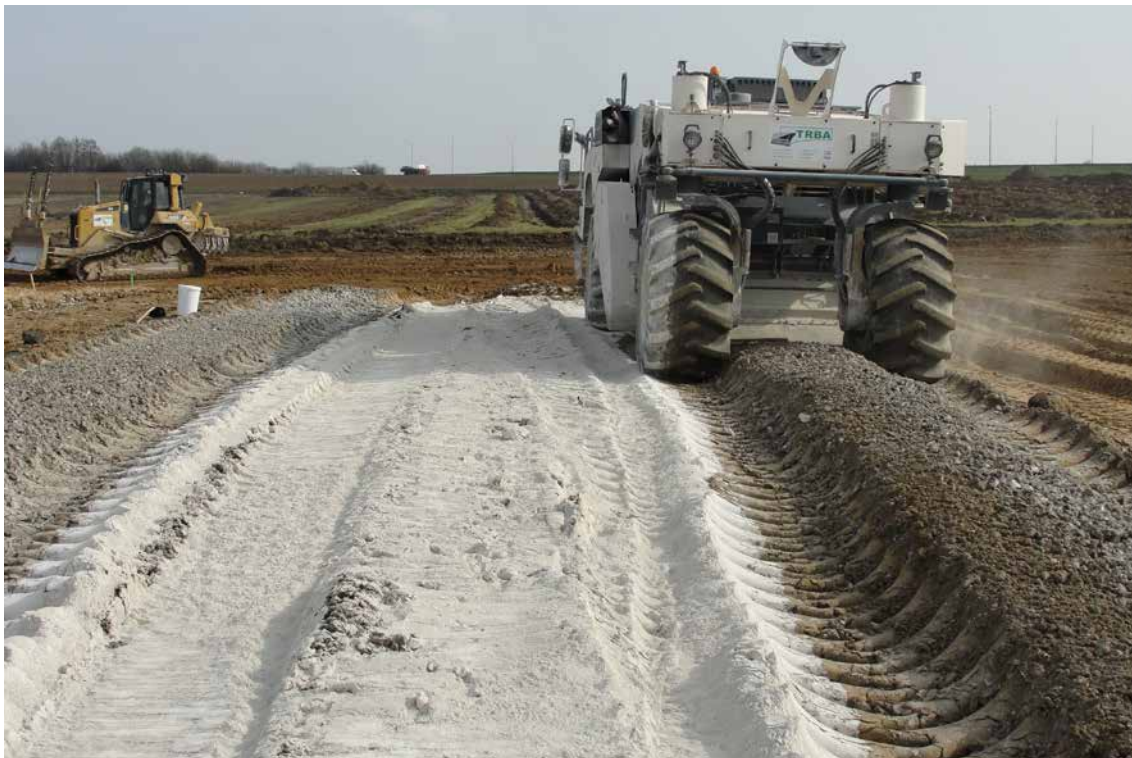
Figure 4.21 – Pulvimixer in action on clay (© Lhoist)
