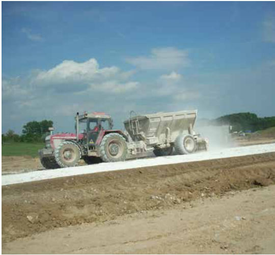
Figure 4.8 – Tractor pulled lime spreading (© Carmeuse)
