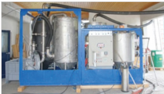
CO 2 scrubber used at the waste water facility at Bad Orb, Germany.
