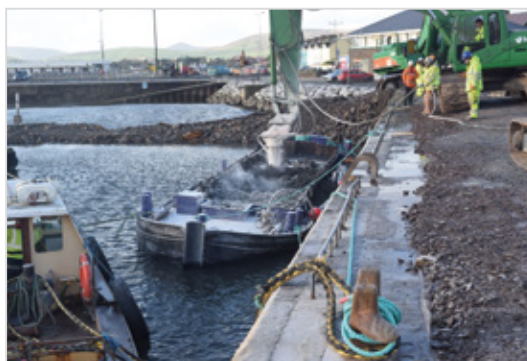
Lime stabilization practice applied on a barge.
