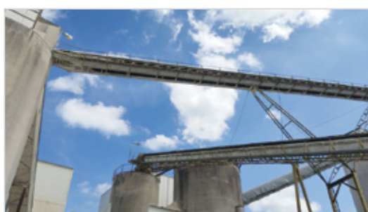
Biofuel tested at Ignaberga in Sweden.
