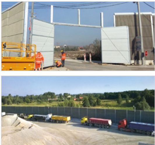
Noise barrier at Miedzianka (Poland).
