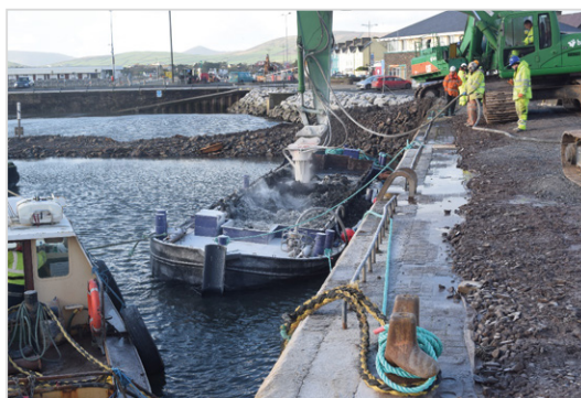
Lime stabilization practice applied on a barge.
